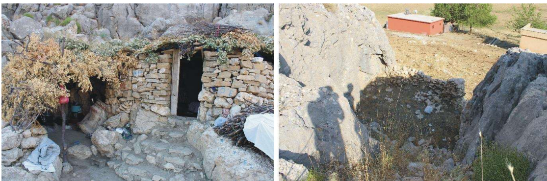
Figure 7. A Hol in Usage (left) and Concrete Houses (July 2016)
